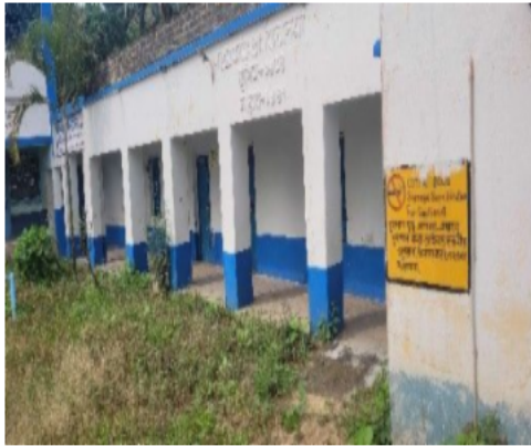
Polling Station Building Front View
