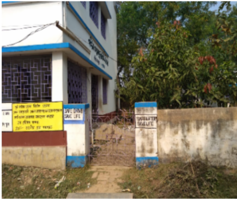
Polling Station Building Front View
