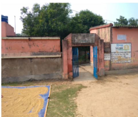
Polling Station Building Front View
