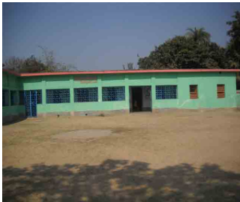
Polling Station Building Front View
