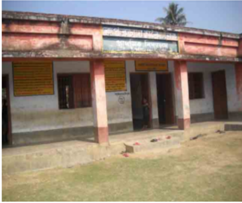
Polling Station Building Front View
