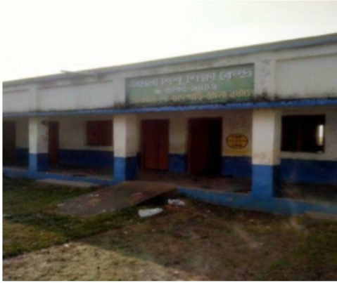
Polling Station Building Front View
