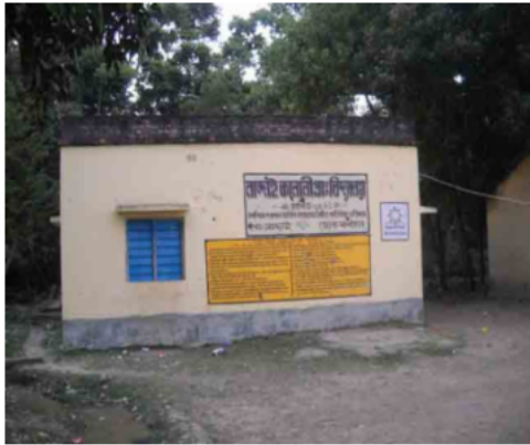
Polling Station Building Front View
