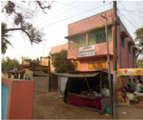
Polling Station Building Front View
