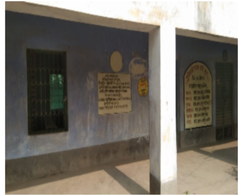
Polling Station Front View
