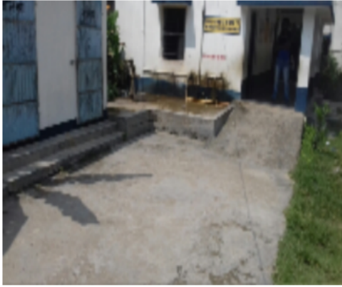
Polling Station Building Front View
