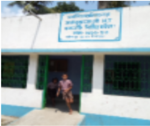
Polling Station Building Front View
