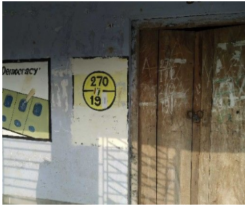
Polling Station Building Front View
