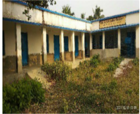
Polling Station Front View
