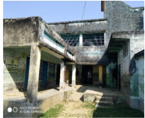
Polling Station Front View
