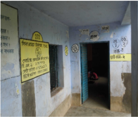
Polling Station Building Front View
