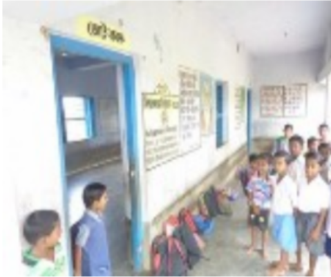
Polling Station Building Front View
