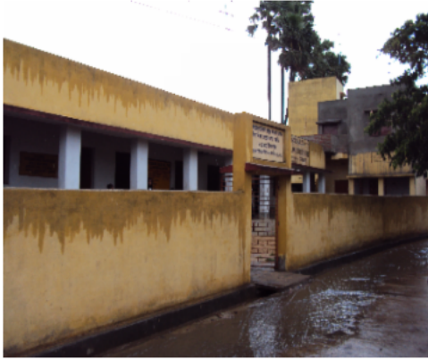
Polling Station Building Front View
