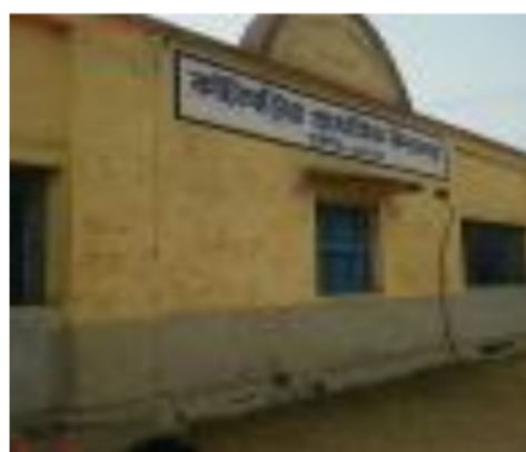
Polling Station Front View
