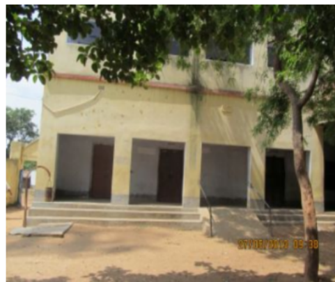
Polling Station Front View
