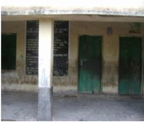
Polling Station Building Front View
