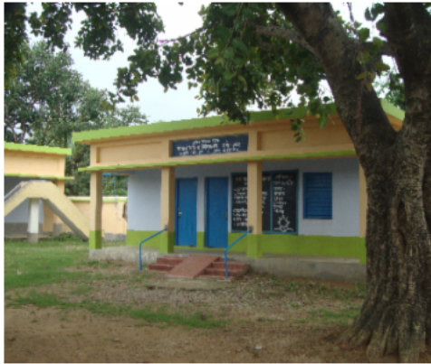
Polling Station Building Front View
