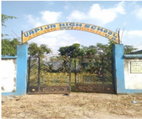
Polling Station Building Front View
