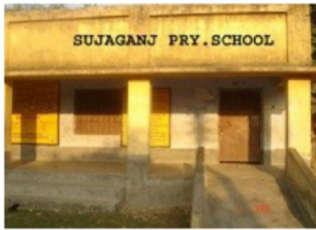
Building Front View
