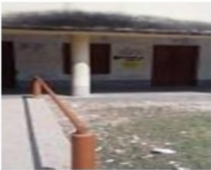
Polling Station Front View
