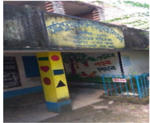
Polling Station Front View
