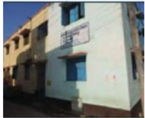
Polling Station Front View
