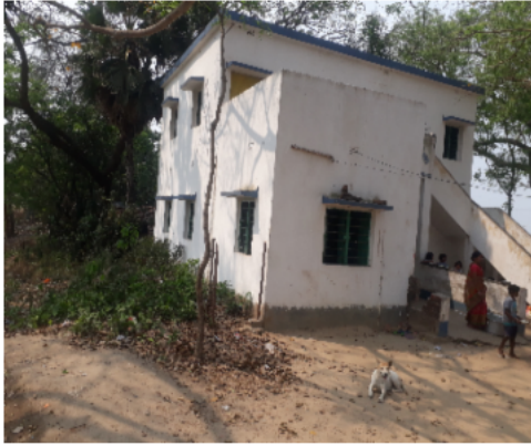
Polling Station Building Front View
