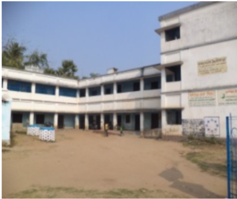
Polling Station Building Front View
