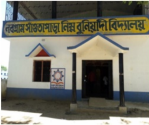
Polling Station Building Front View
