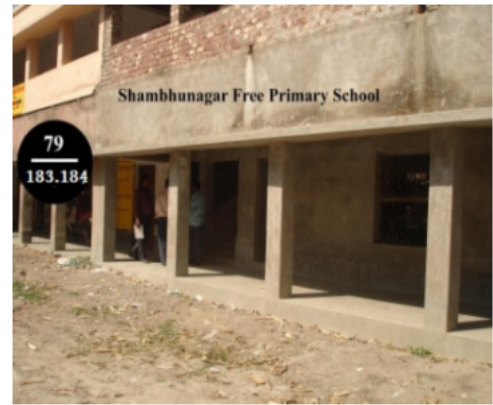
Polling Station Front View
