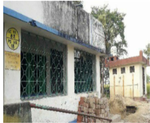
Polling Station Front View
