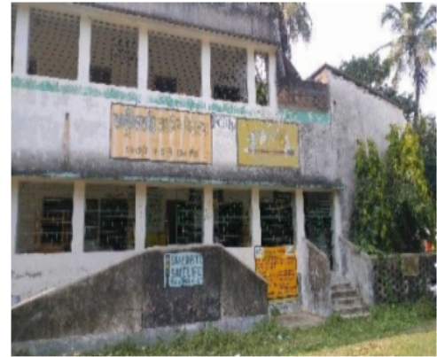
Polling Station Front View
