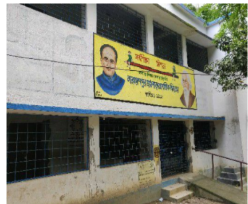
Polling Station Front View
