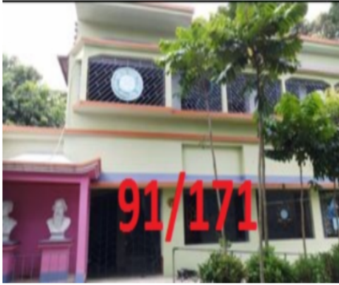
Polling Station Building Front View
