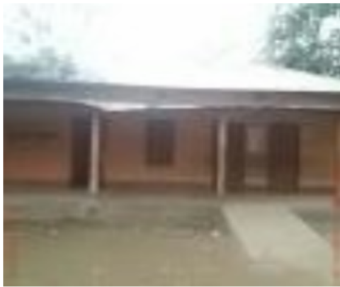
Polling Station Building Front View
