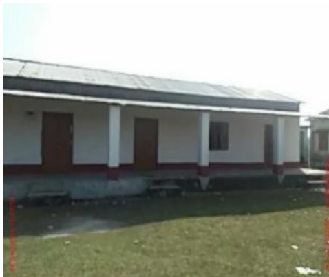
Polling Station Building Front View
