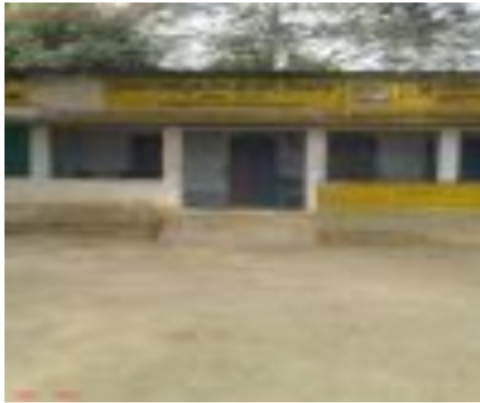
Polling Station Building Front View
