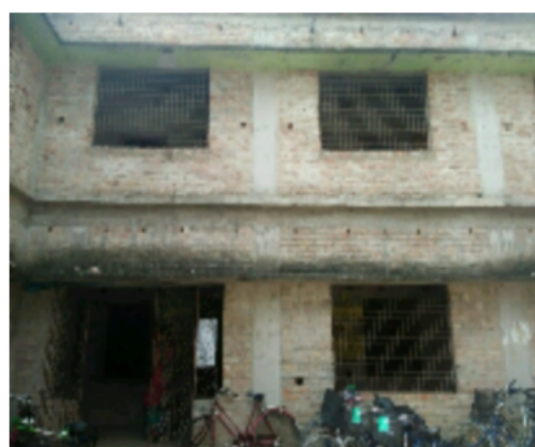
Polling Station Building Front View
