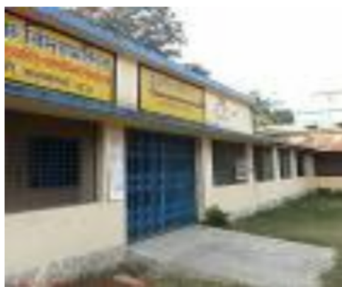
Polling Station Building Front View
