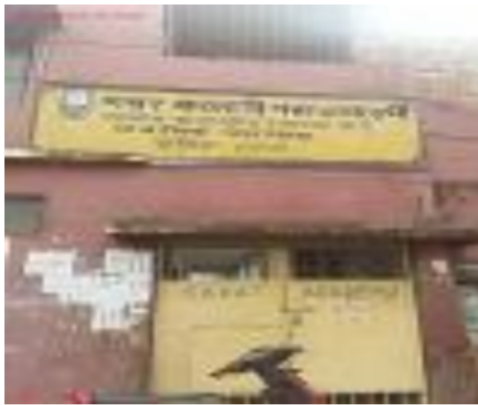
Polling Station Building Front View
