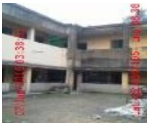
Polling Station Building Front View
