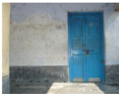
129/164 - Bhuban Khali No. 4 F.P. School
