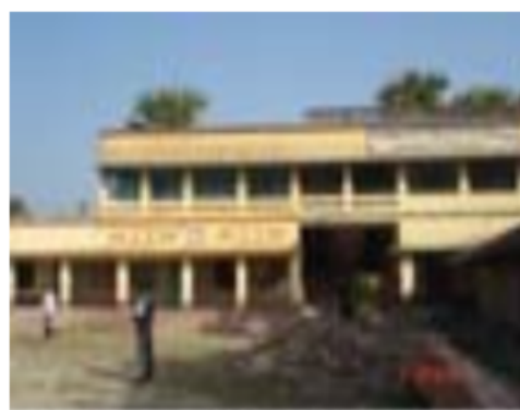
12902 - Paschim Bahduta F.P. School (Room No. 1)
