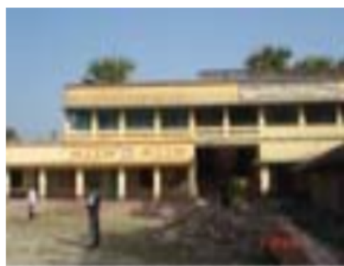
12902 - Paschim Bahduta F.P. School (Room No. 1)
