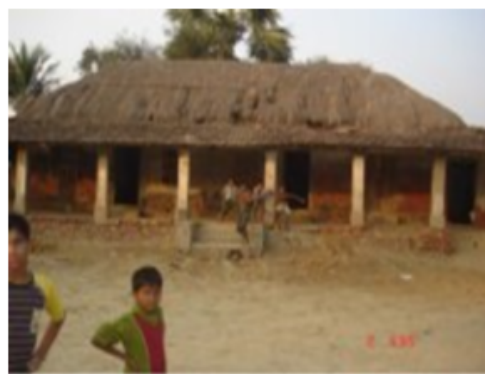
129/89 - Gopinagar Kalikapur Kachhari Bari Medical Sub-Centre
