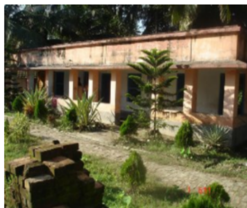
Polling Station Building Front View
