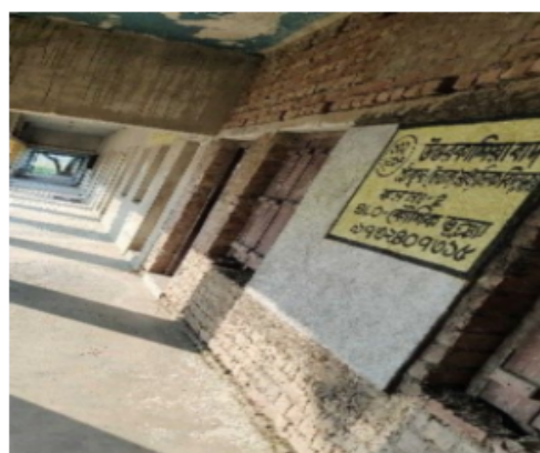
Polling Station Building Front View
