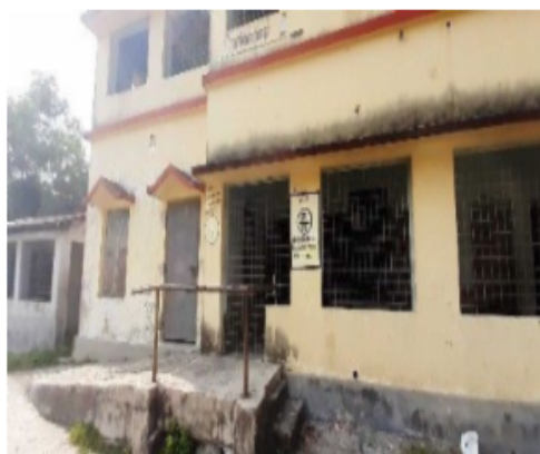
Polling Station Building Front View
