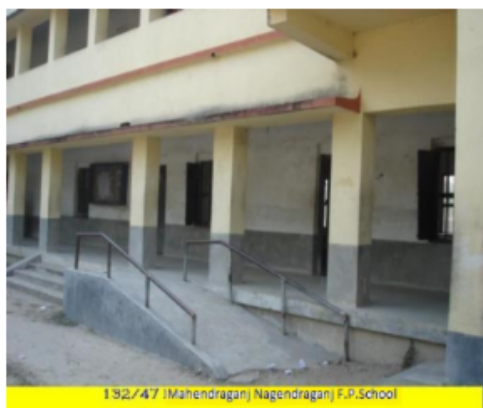
132/47 | Mahendraganj | Nagendraganj | F.P. School
