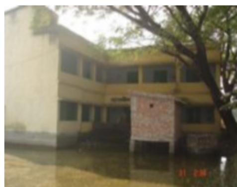
136/139 - Moydah F.P. School (Room No. 1)
