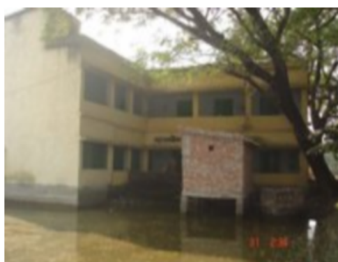
136/139 - Moydah F.P. School (Room No. 1)
