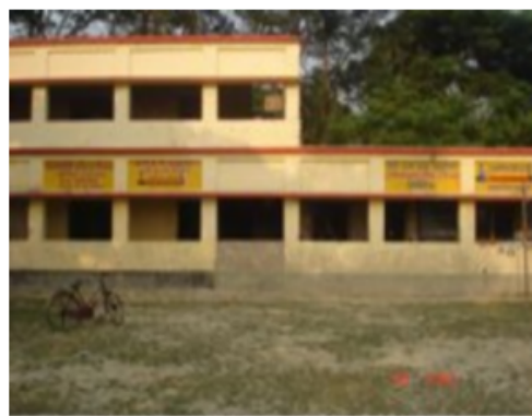
136/149 - Mayahouri F.P. School (Room No. 1)
